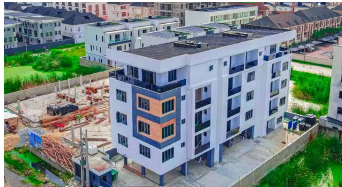
CAMBERWALL ADVANTAGE 1 COMPLETED AND DELIVERED
