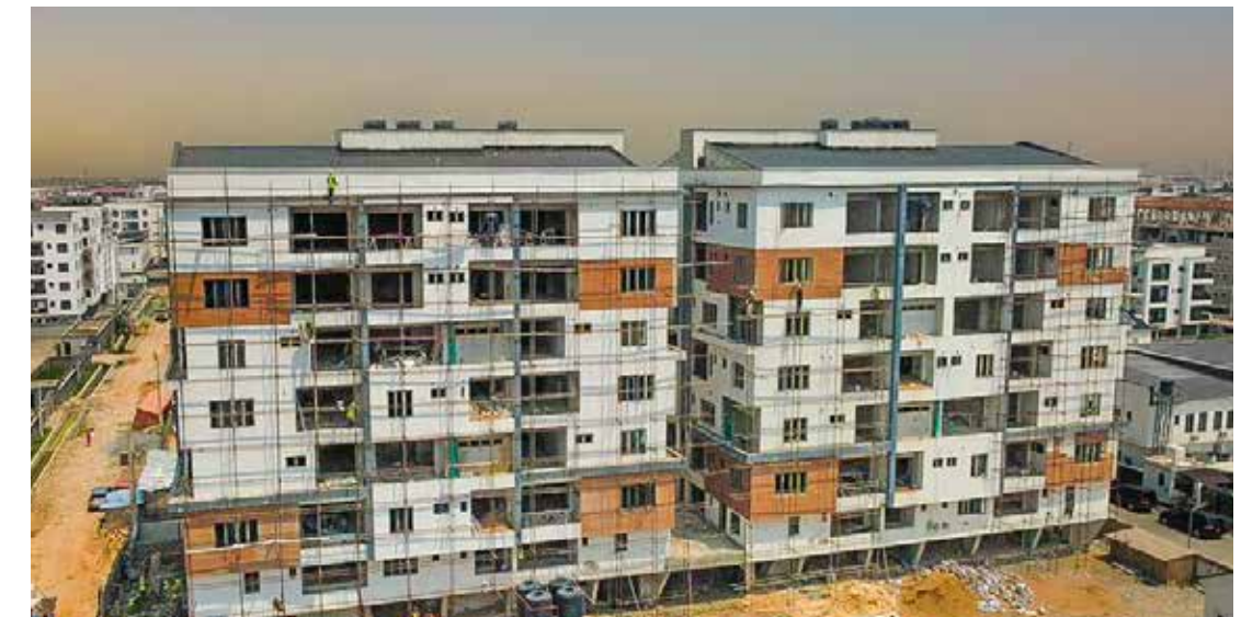
CAMBERWALL ADVANTAGE 3 CONSTRUCTION ONGOING
