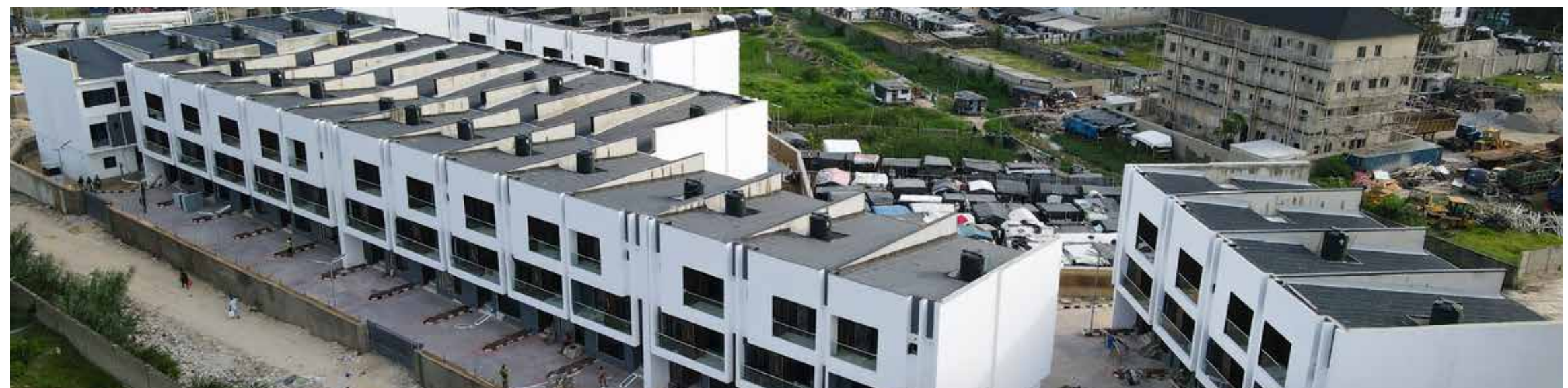
CAMBERWALL ADVANTAGE 5 COMPLETED AND DELIVERED
