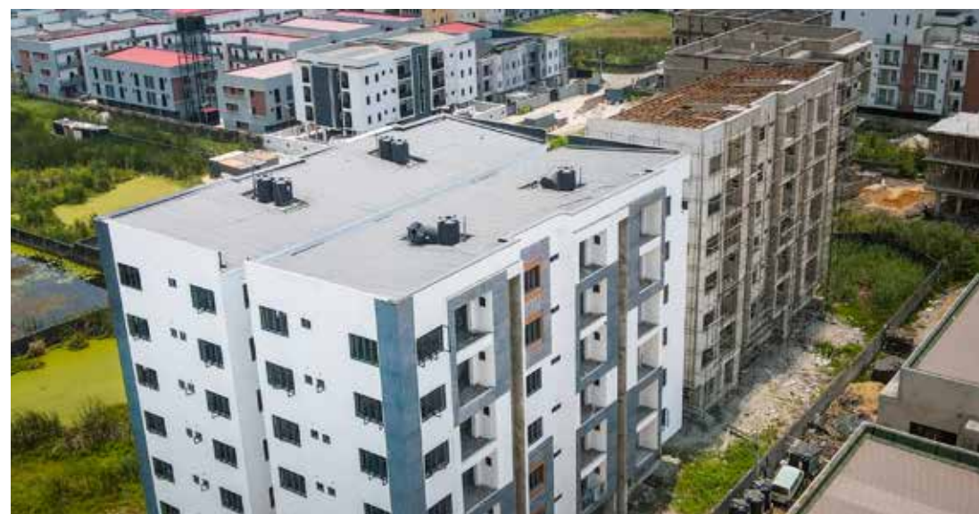
CAMBERWALL ADVANTAGE 4 CONSTRUCTION ONGOING
