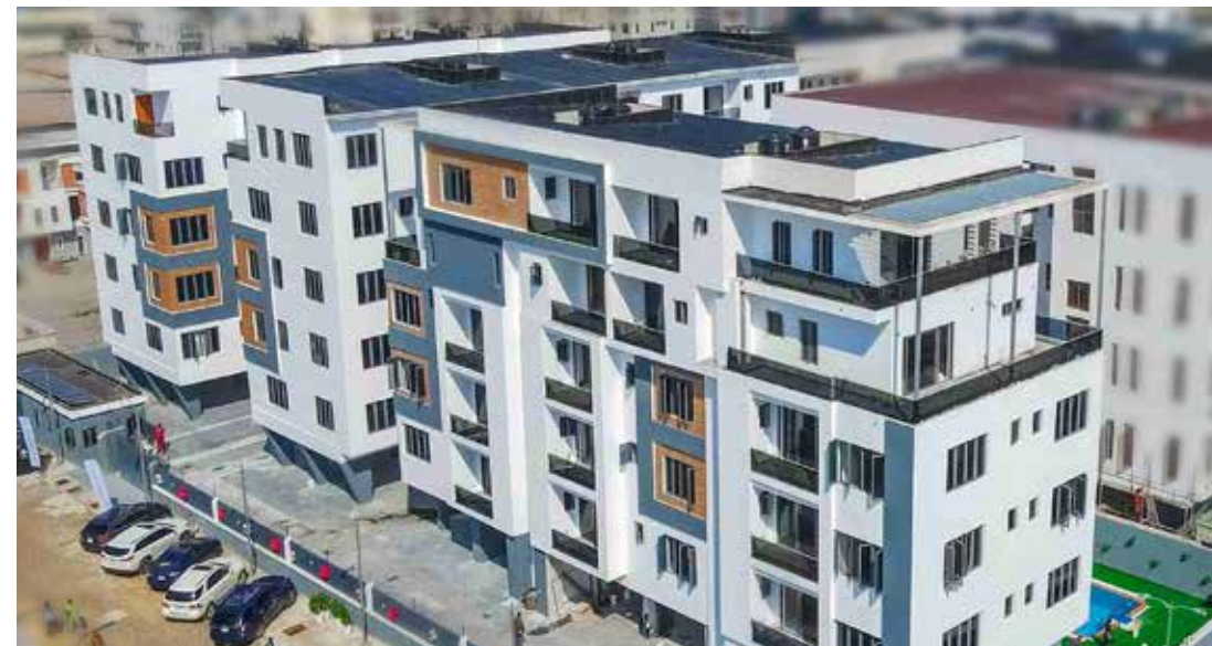
CAMBERWALL ADVANTAGE 2 COMPLETED AND DELIVERED
